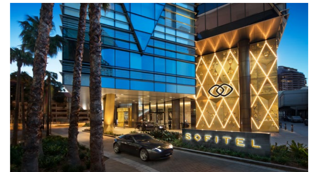
Sofitel Sydney Darling Harbour exterior
